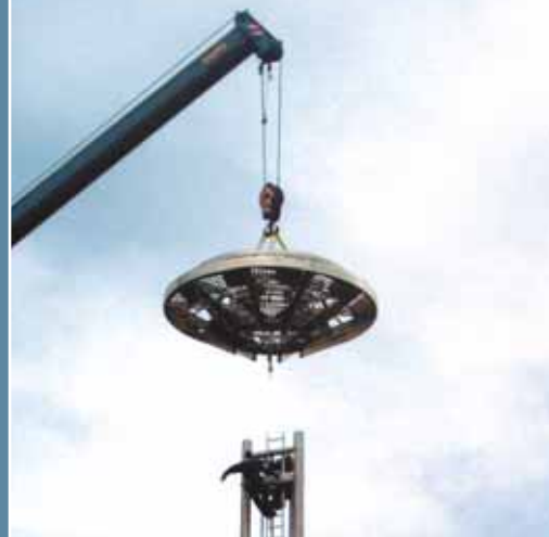
HIGH MASTS INSTALLATION
