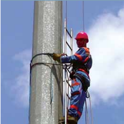
HIGH MASTS MAINTENANCE
