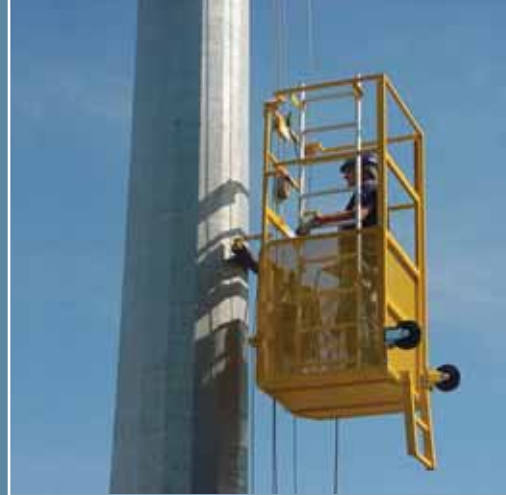
HIGH MASTS AND ACCESSORIES RESTORATION
