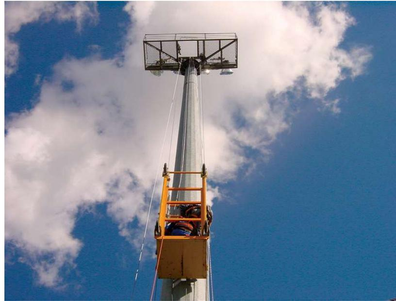
ACCÈS AUX PROJECTEURS CLASSIQUE PAR ECHELONS/CÂBLE ET ÉQUIPEMENT INDIVIDUEL DE SÉCURITÉ INSTALLATIONS PERMANENTES (PALIERS DE REPOS, PASSERELLE, ÉCHELLES...)
